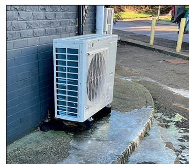
USING THE SOAK-AWAY PREVENTS THE CONDENSATE FROM FLOWING ONTO PATHS AND FREEZING - CAUSING A SLIP HAZARD.
